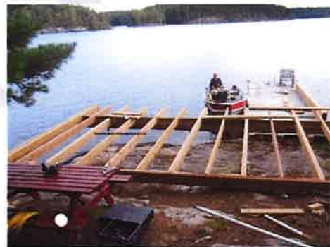
Figure 5 Example of Wood Decking Construction.
