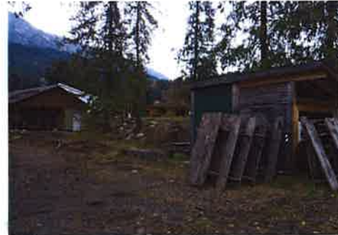
Figure 1 Existing Buildings at Lakeside Campground.
